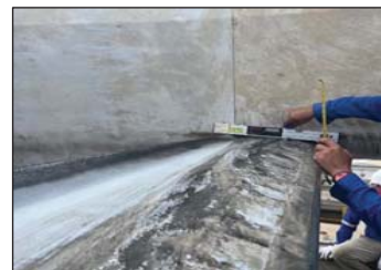
Pict. 5 Measure Tip track, Blade tip clearance, and Blade pitch angle before.
