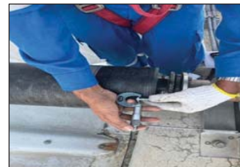
Pict. 8 Check coupling gap after final alignment.
