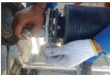
Pict. 3 Check coupling gap before dis-connect drive shaft.
