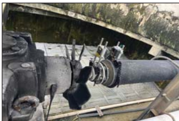
Pict. 2 Check drive shaft alignment gearbox before.
