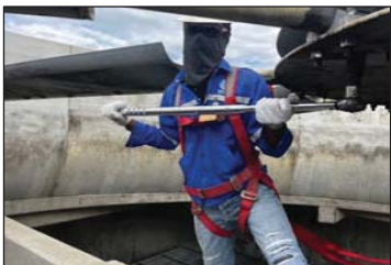
Pict. 12 Tighten torque bolt of fan blade.
