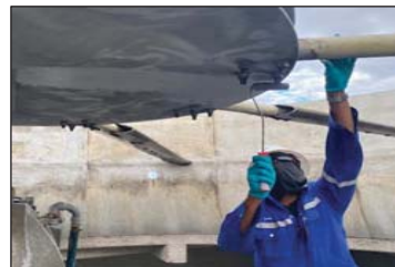
Pict. 16 Coating on hub fan blade.
