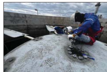
Pict. 13 Tighten torque bolt of hub plate.
