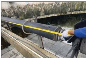
Pict. 4 Check distance between shaft ends before dis-connect drive shaft.
